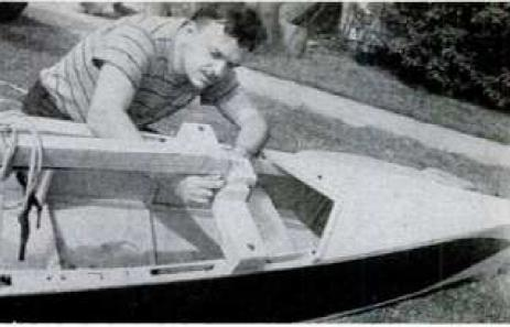
Main hull presents trim appearance as it nears completion (left). Note the large screw eyes in stern. A pin dropped through these and two mating eyes in the rudder hold rudder-tiller
