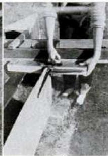
Two hinges bolted together join the boom and mast (left), allowing the boom vertical and horizontal movement. A plastic drink stirrer (center) serves as shear pin for the rudder.
