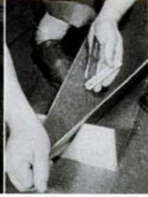
Glued frames for the main hull are spaced at 24" intervals along keel (above left). Guide cuts for beveling the keel and chines are made with a saw (center). Battens are clamped to
